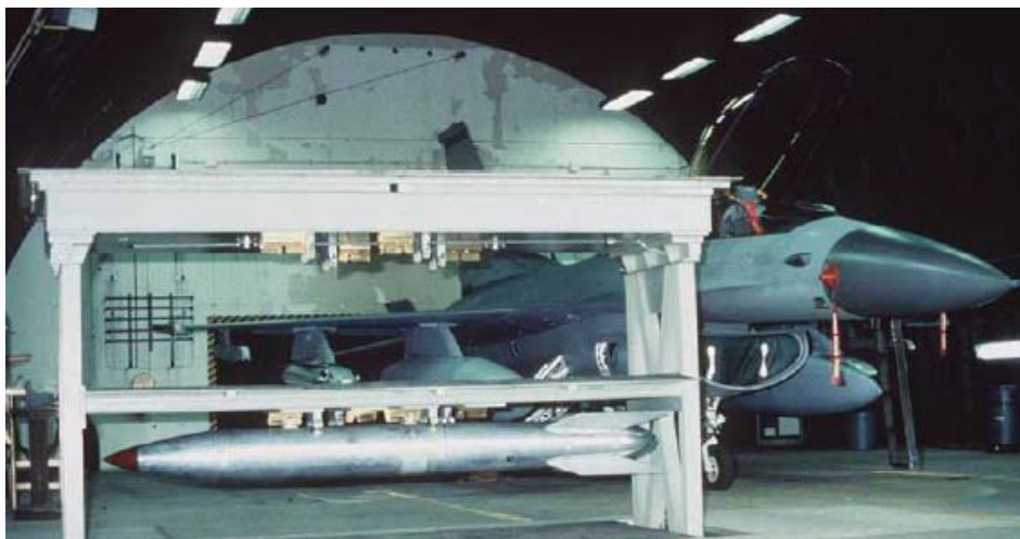
Elevated Weapons Storage Vault (WSV) with B61 body in Protective Aircraft Hangar. Source: U.S. Nuclear Weapons in Europe: A review of post-Cold War policy, force levels, and war planning. Hans Kristensen, NRDC.
